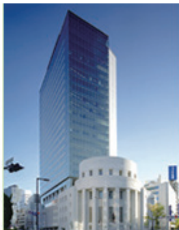
Osaka Securities Exchange Bldg.
