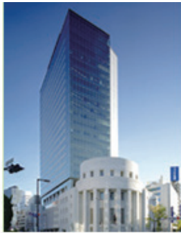
Osaka Securities Exchange Bldg.
