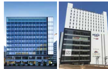
Ichibancho Heiwa Building Solala Plaza
