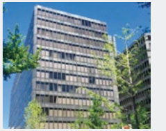
Osaka Midosuji Building (Osaka City)
