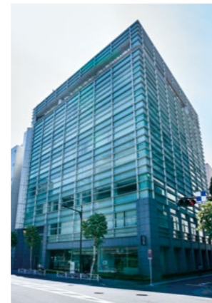
Kabutocho Heiwa Building No. 6 (Chuo-ku, Tokyo)
