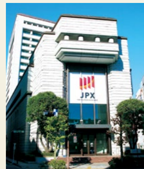
Tokyo Stock Exchange Building (Tokyo)
