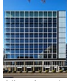
Ichibancho Heiwa Building
