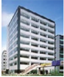
Shimbashi Square Building
