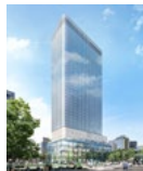
SAPPORO ONE (acquisition of ZEB Oriented certification)
