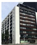
Heiwa Real Estate Nagoya Fushimi Building
