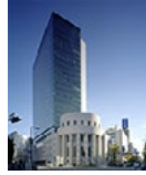
Osaka Securities Exchange Bldg.
