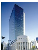
Osaka Securities Exchange Bldg.
