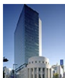
Osaka Securities Exchange Bldg.
