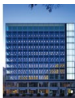
Ichibancho Heiwa Building
